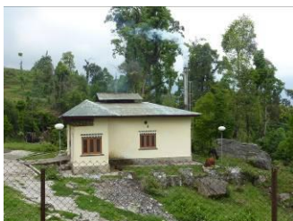
Figure 19: Alikha incinerator in Gedu Town
