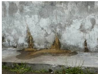
Figure 10: Sign of wear in one of the oxidation ditches
