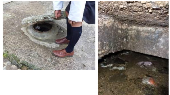
Figure 7: Issue with overload septic tanks and illegal dumping of untreated wastewater
