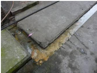
Figure 14: Grey water discharged in house drain
