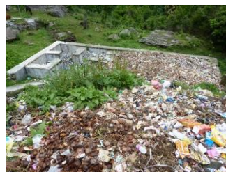
Figure 20: Overloaded receiving ramp
