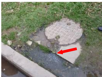
Figure 3: Septic tank overflow
