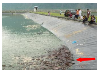
Figure 12: Maturation pond at Phuentsholing Sewage Treatment Plant
