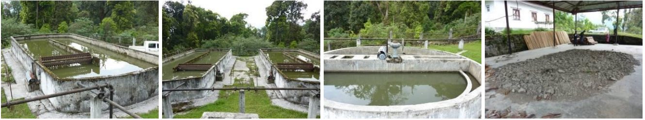
Figure 9: Sewage treatment plant in Gedu
