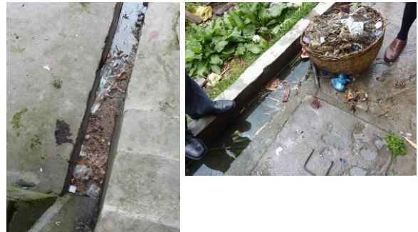
Figure 15: House drains blocked by garbage
