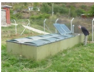
Figure 13: Eco-line Sewage Treatment Plant in Thimphu
