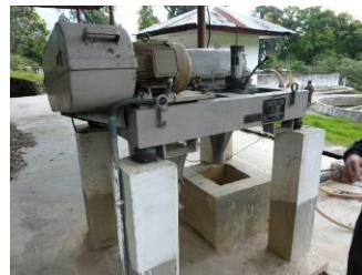
Figure 11: Broken equipment (dewatering machine)
