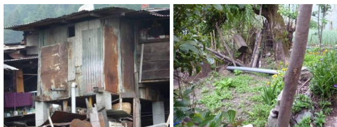
Figure 4: Improper wastewater discharge from toilet
